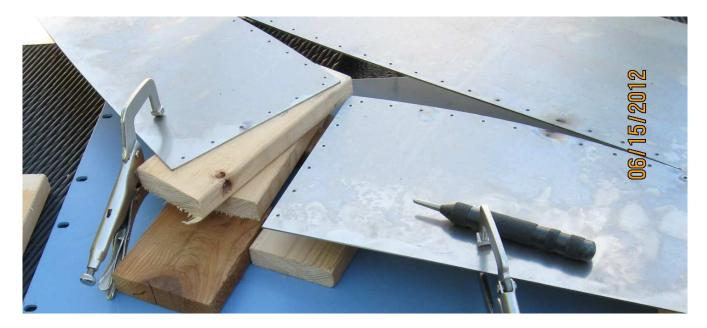
Transferring holes with auto center punch from one pattern to another. I forgot that I had set of transfer-punches (you just need to choose the one which perfectly fit to original hole).
