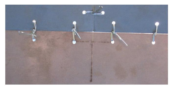
This picture just shows twisted wire connection. Seams fitting looks much better because of stronger pull. The joint is exactly where it suppose to be according laser's mark.
